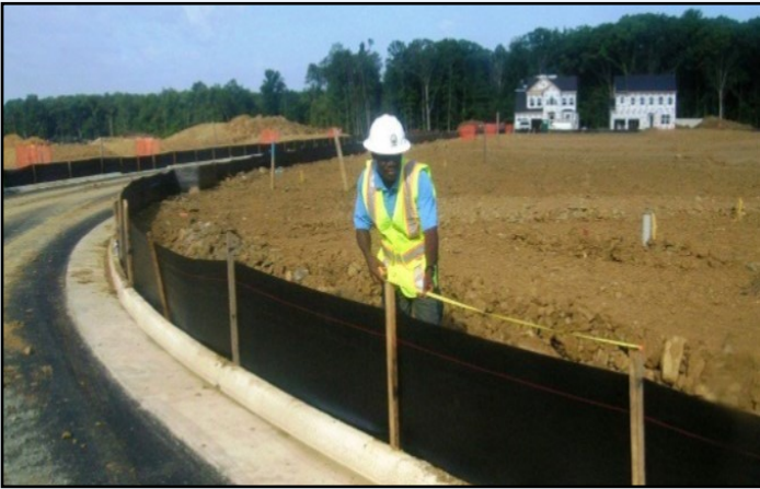
Photo: Silt Fence Installation
