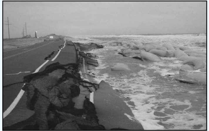
Photo: Storm damage along NC 12
